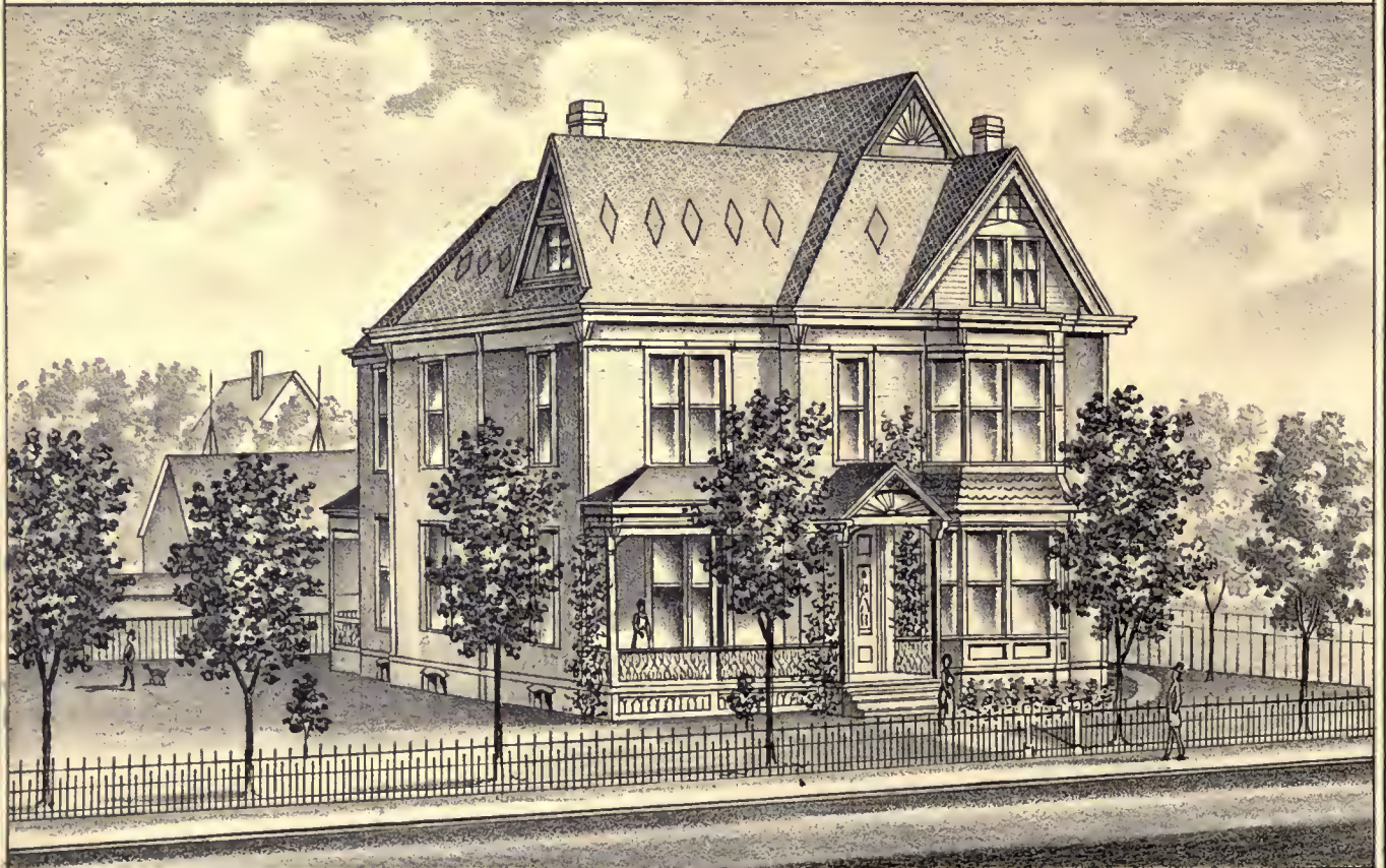
RESIDENCE OF F. W. LOWENTROUT, 603 MARKET ST., BLOOMINGTON, ILL.
