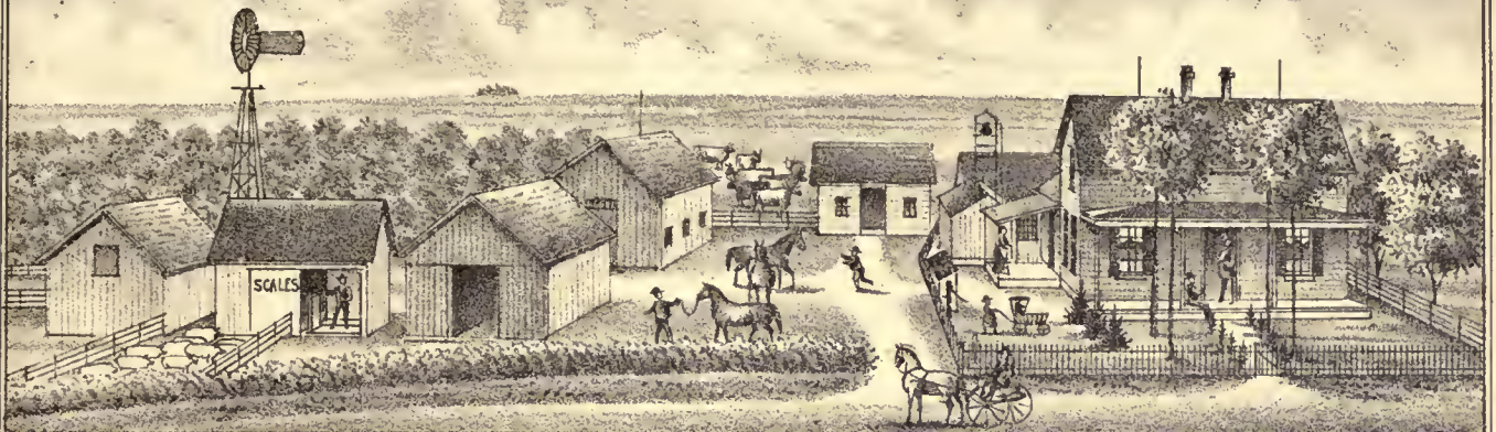
RES. OF ARTHUR S. CATRON, SEC. 25, TOWANDA TOWNSHIP.
