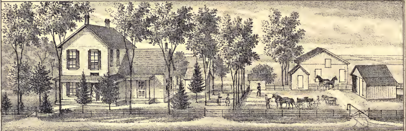
RESIDENCE OF JOS. T. MARTIN, SEC. 1, (T. 21), RANDOLPH TOWNSHIP.
